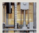
Front fiberglass tower panel removes for easy service access to all mechanical and electrical components.
